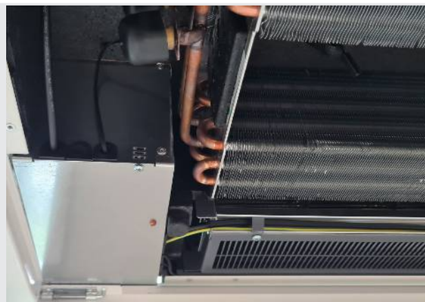
Position of electrical junction box (with condensate tray removed)
