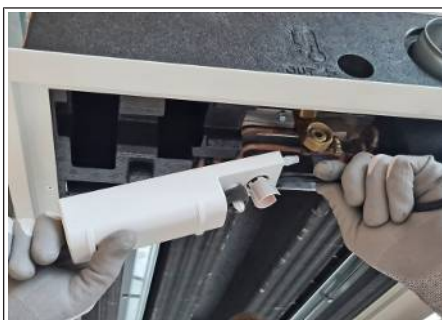
Fig. 44: Dismantling the condensate pump
