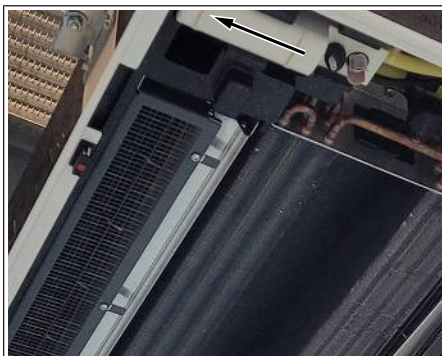
Fig. 22: Correct position of the condensate pump
