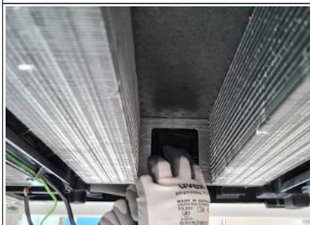
Fig. 25: Removing the primary air cover
