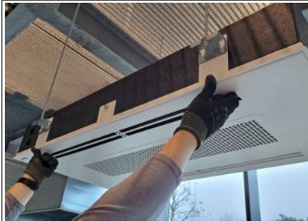
Fig. 7: Opening the design panel
