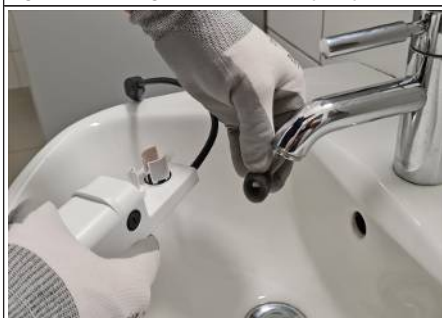
Fig. 46: Cleaning the dirt filter
