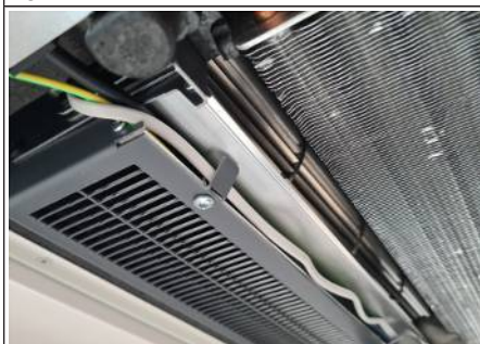
Fig. 19: Routing the actuator cable
