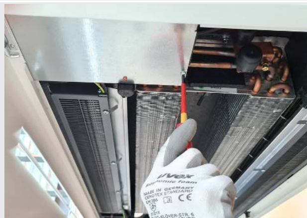
Use a Phillips screwdriver to open the electrical junction box and remove the cover of the junction box.
