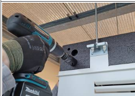
Fig. 16: Opening up the connection holes
