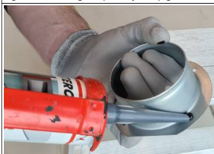
Fig. 24: Sealing the primary air connection spigot
