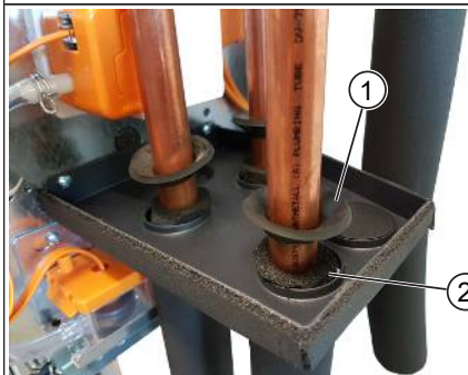
Fig. 18: Gluing rubber pipe collars with insulation
